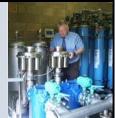
**River, Canal and Stream Supplies** - Filters used for cooling, potable and process water. TC Filters are available for any flow at any micron to remove silt and other debris found in surface water which can then be fed into a system or onto further fine filtration. The use of our filters can help protect heat exchangers as well as other cooling systems.
