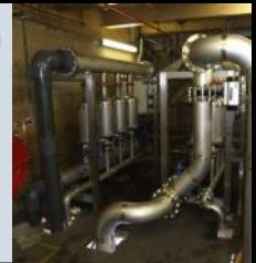
**Final Effluent and waste water** - The ability to remove particles allows water to be re-used and so saves on mains water. Waste water can be cleaned sufficiently to either re-use it or clean enough to achieve required cleanliness.
